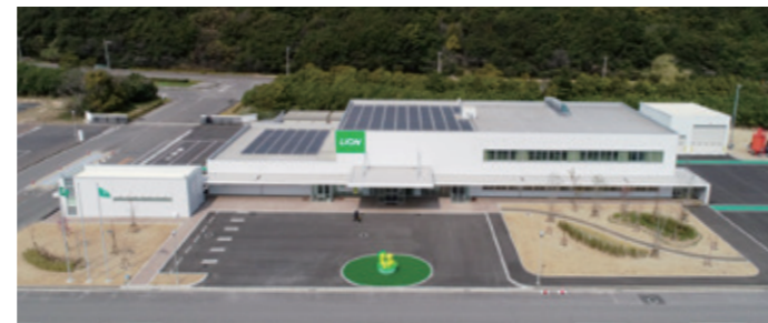
Solar panels on the roof of the employee facility building
