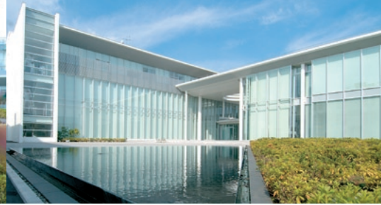
The triangular pond uses rainwater
