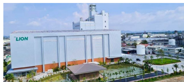
The new spray-drying tower building at LCT
