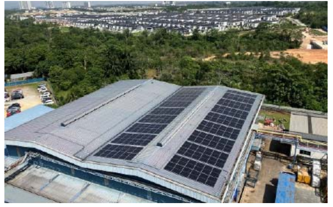
Exterior view of the SL warehouse
