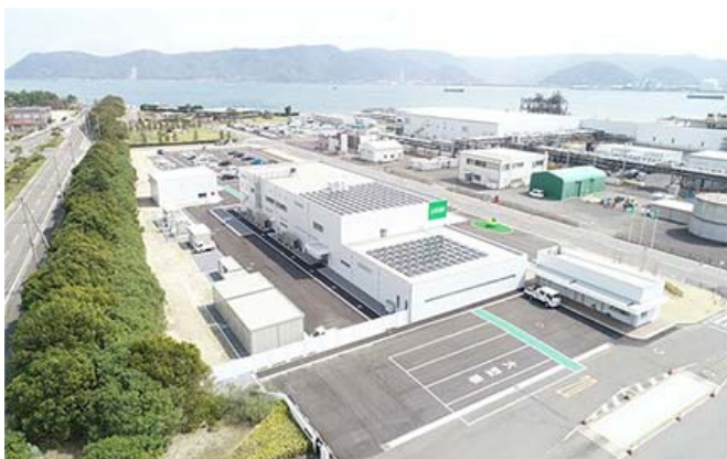
Lion Chemical Co., Ltd. New welfare building at the Oleochemical Plant (Sakaide)
